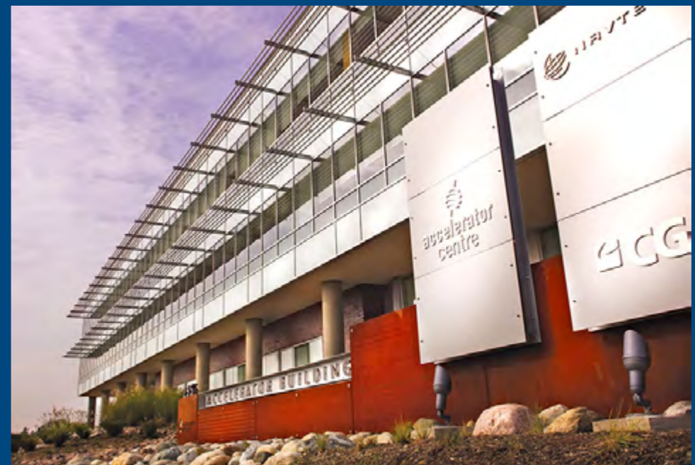
ACCELERATOR CENTRE - WATERLOO
